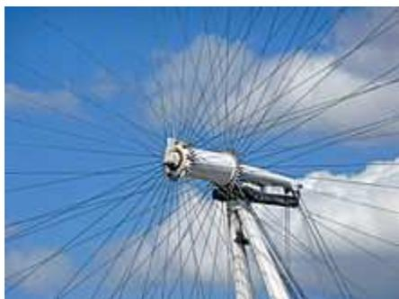
The spindle, hub, and tensioned cables that support the rim
